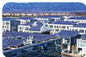
屋顶光伏 Roofing Solar
