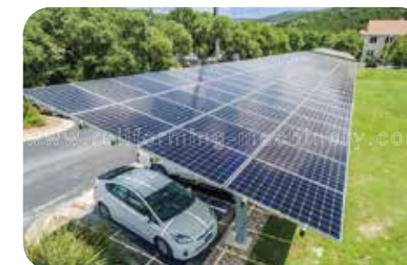
车棚光伏 Carport Solar
